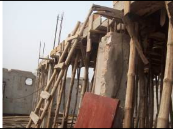
4 th floor under construction
